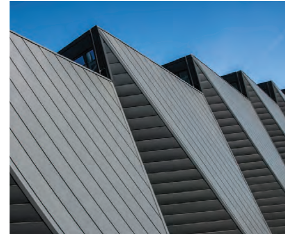
Figure 3: Materials Source: Dezeen, Switchgear Station, C.-F. Møller
