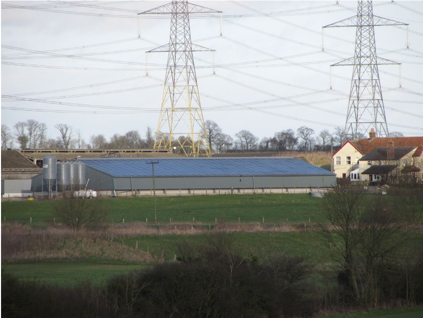
Figure A2.3 Large scale farm building with solar roof
