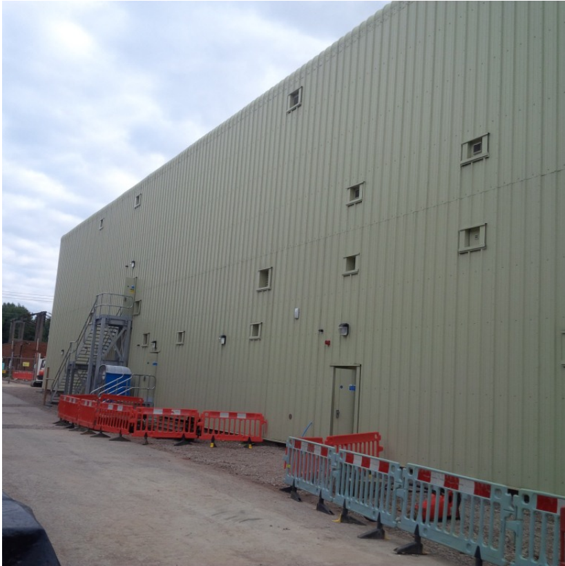
Figure A2. 5 Gas insulated Substation building clad in metal sheet
