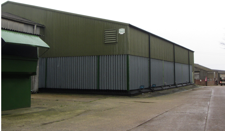
Figure A2.1 Contemporary barn building clad in metal sheet
