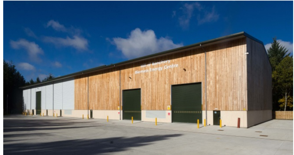
Figure A2.4 Biomass centre with wooden cladding
